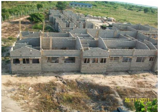
Inpatient ward currently under construction
